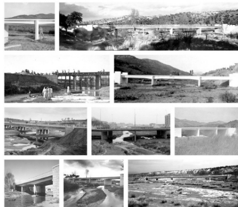
Collection of images of different bridges of the CPAE. Source: Carlos Fernández Casado Fond, CEHOPU-CEDEX.
