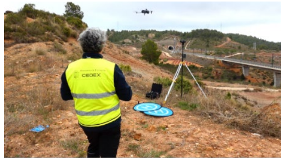
Drone-based operations for obtaining the point cloud of the viaduct
