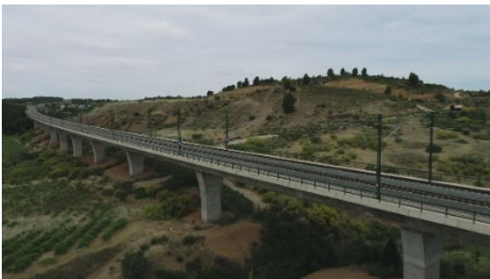
Instrumented Viaduct for the ERJU Project
