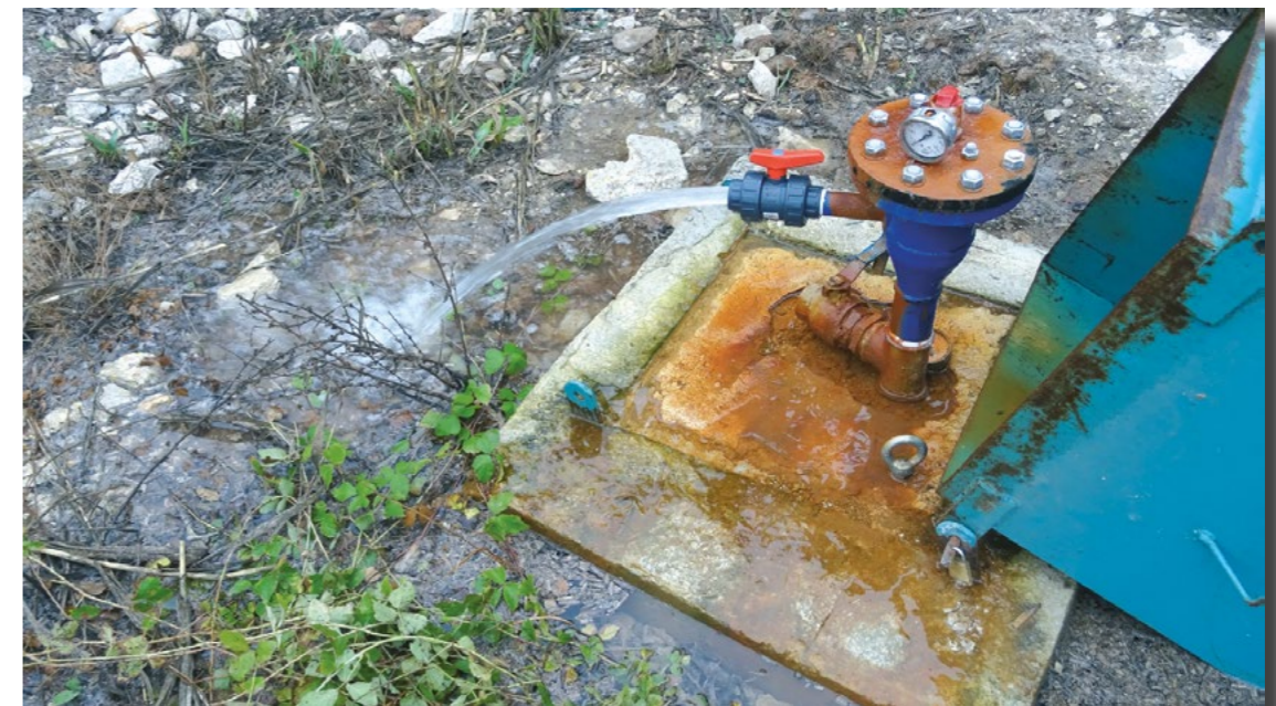
Upwelling borehole used as a piezometer and sampling point located in an aquifer downstream of the Bellús reservoir.
