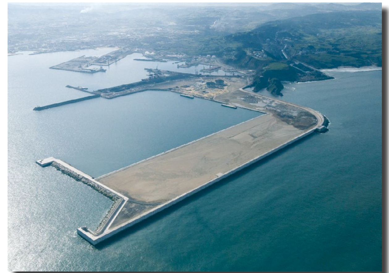
Figure 5. Project for railway access to the north quay (port of Gijón). Aerial view of the quay.
