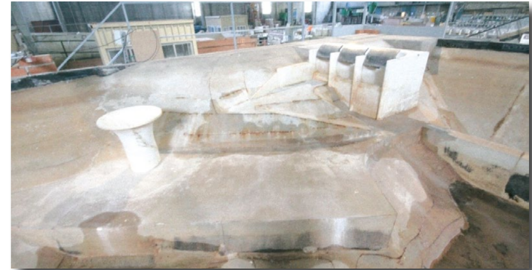
General view of the Yesa landfills with the variant solution.
