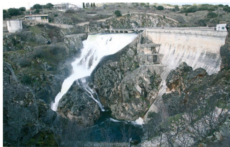
Spillway of the El Villar Dam.
