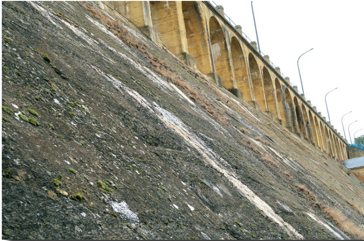
Study of the Villameca dam.
