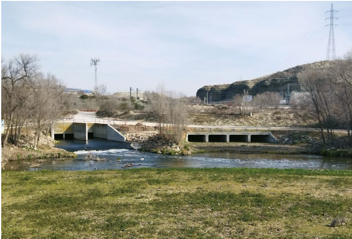
Spillways of the La Gavia WWTP and La Gavia stream, on the left bank of the Manzanares river.
