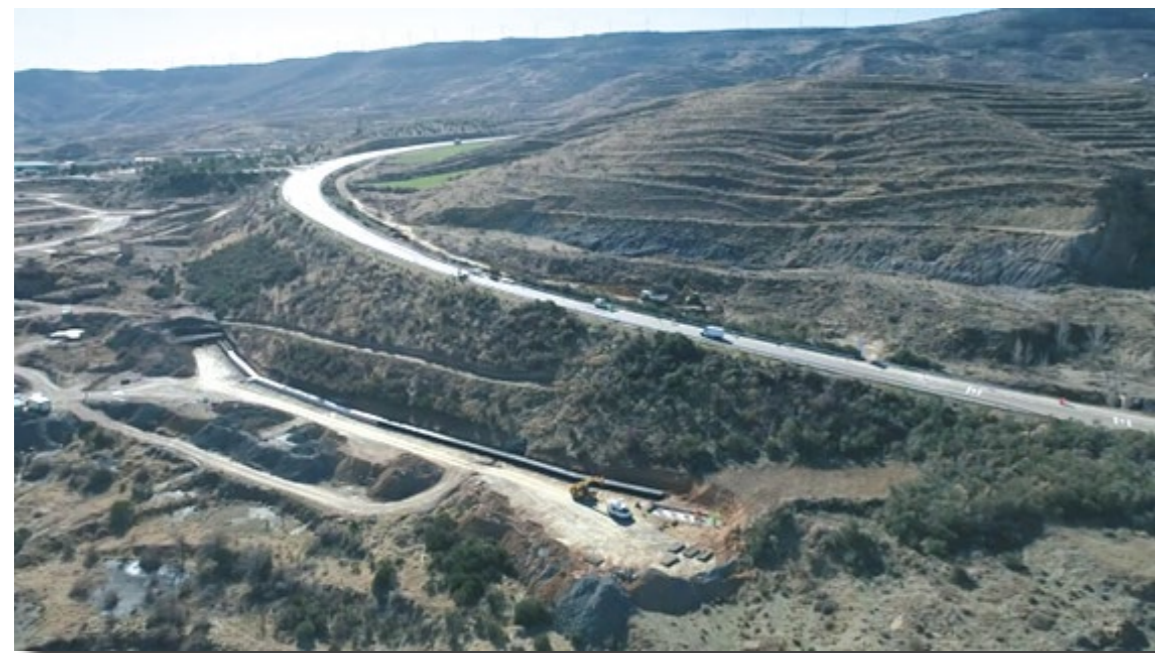
View of the section of the N-420 with geotechnical pathology.
